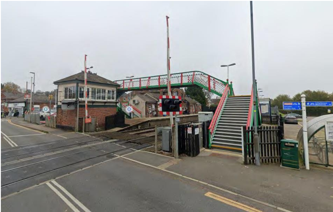
Figure 2.1 Narborough level crossing
